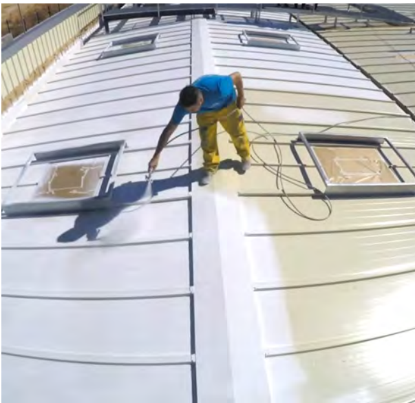
Picture 8 - Application of SurfaMix Universal Primer
