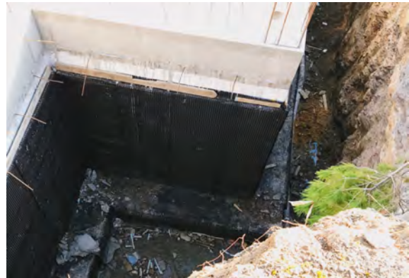
Picture 4 - Basement Insulating system before landfilling
