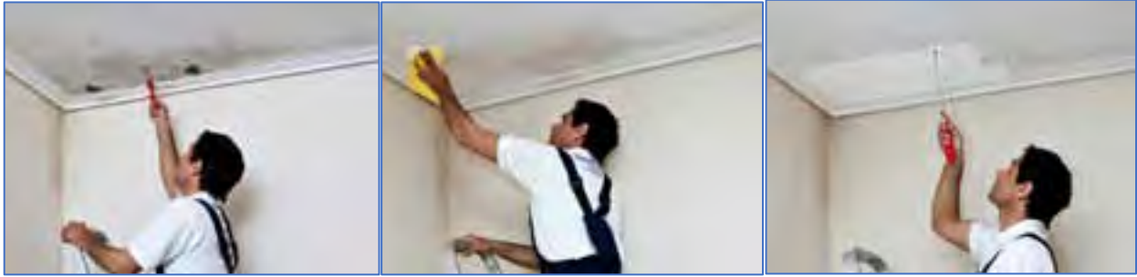
Picture 16 – Mould removal and painting sequence by DeSalin AM and SurfaPaint AquaX
