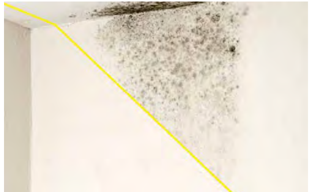
Picture 18 – Application of DeSalin AM on a mouldy wall
