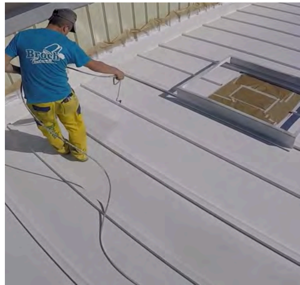
Picture 9 - Application of SurfaPaint ThermoDry Elastomeric Roofs on primed surface
