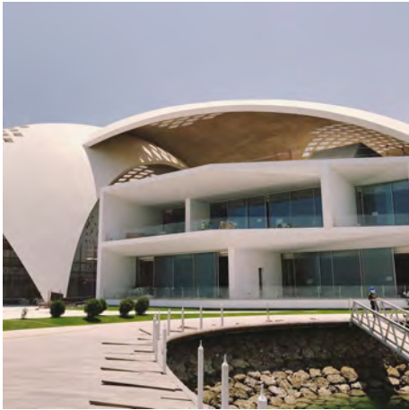
Picture 82 - Dust pick-up underneath a dome, subjected to desert and seawater environment
