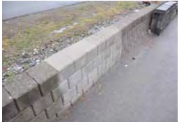
Picture 106 – The effect of SurfaShield CX in the fungi-rich environment of Norway, six months after installation
