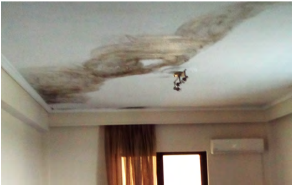
Picture 17 – Real life example of a ceiling cleaned with DeSalin AM (clean, bottom right) and bleach solution (upper left, mouldy) after a 2 years period
