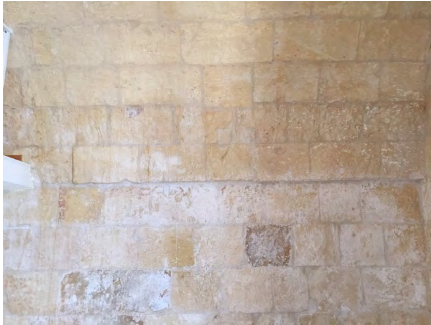
Picture 42 – Soft stone stabilization substrate after application of SurfaPore FX WB (upper half). Dusting and deterioration have stopped.
