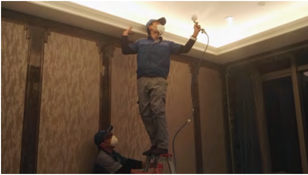
Picture 63 - Application of SurfaShield C on painted ceiling
