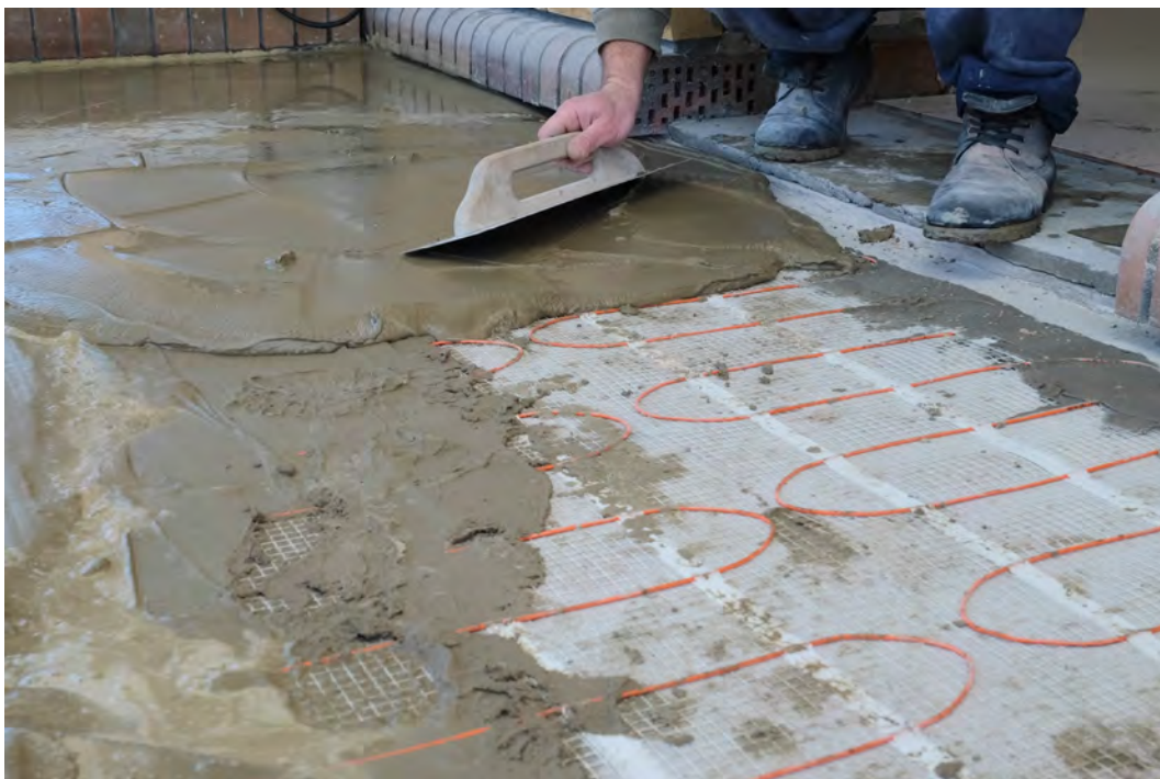
Picture 140 - High thermal conductivity cement encasing of underground floor heating system, which is supported on FeatherPlast PT400
