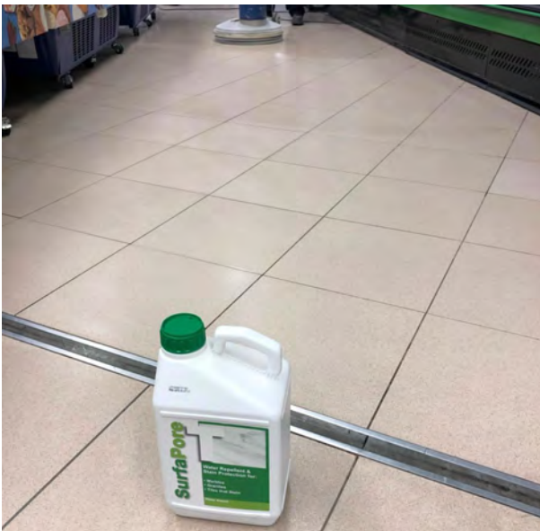
Picture 21 - Application of SurfaPore T on Grès Porcellanato tiles
