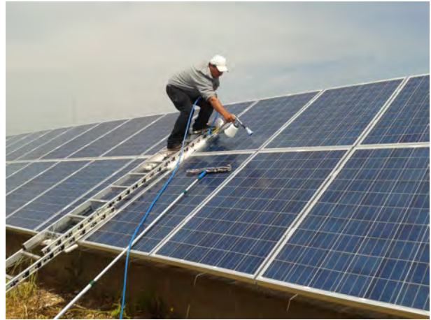
Picture 27 - Application of SurfaShield G on pre-installed panels
