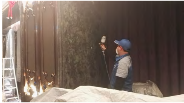
Picture 64 - Application of SurfaShield T on vertical marble surface
