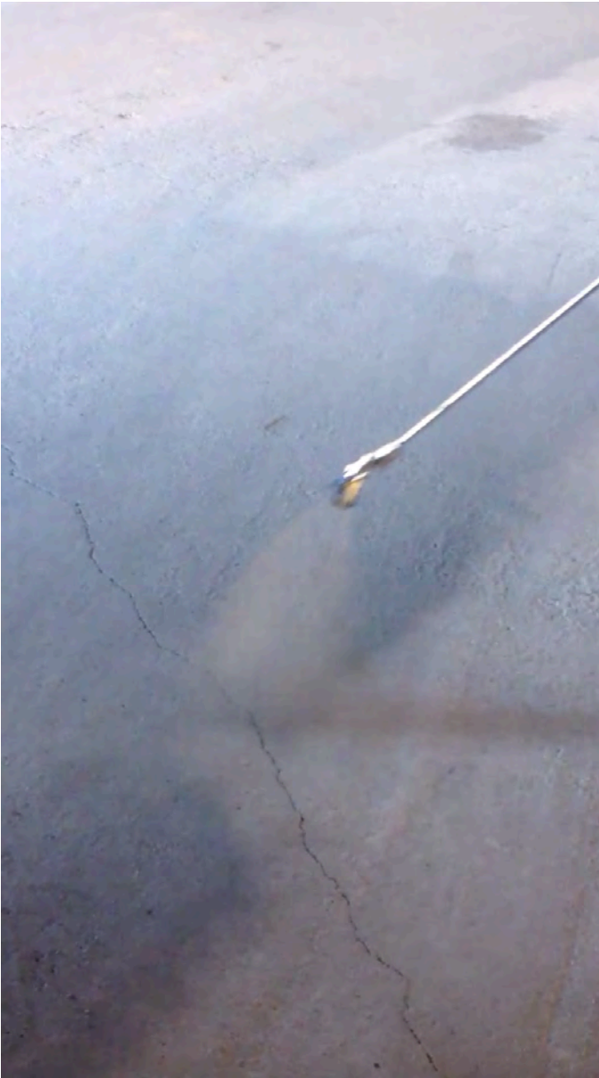
Picture 89 - Application of SurfaPaint Floor paint on a warehouse cement floor
