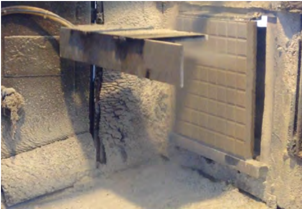
Picture 105 – Industrial application of SurfaShield CX on pavement slabs
