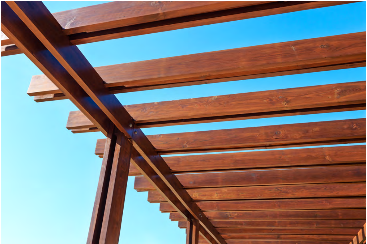
Picture 92 - Wood pergola treated with SurfaPaint Wood Stain and SurfaPaint Wood Varnish - UV Blocker five years after application under Mediterranean sun, next to Mediterranean Sea
