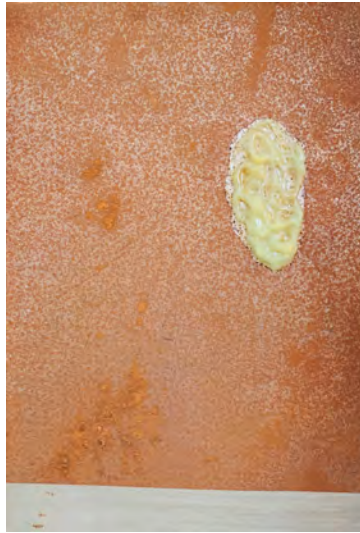
Picture 133 - Application of DeSalin Rust Remover on a vertical metal surface
