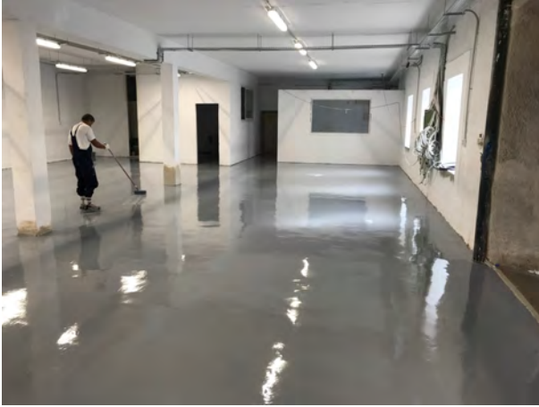
Picture 37 - Application of EPFNova Solvent-Free, Epoxy Floor Top Coat
