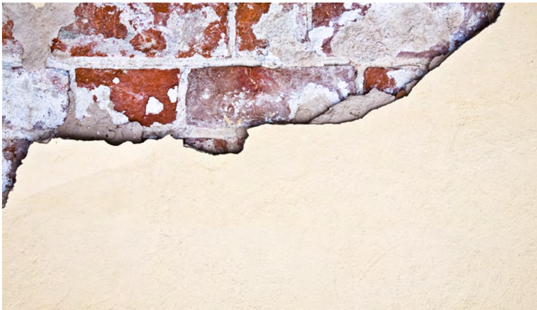
Picture 103 - Performance comparison of weathering effect between SurfaMix C (lower part) and a Latex SBR render (upper part) after three years exposure in Mediterranean environment.
