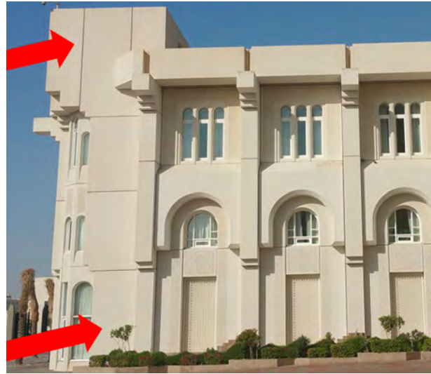
Picture 142 - A palace made of cementitious rendering. The rendered façade appears yellowish on the upper part, while cleaned and fresh in the lower part, as of intense maintenance & cleaning efforts.
