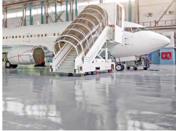
Picture 38 - Application result of Nova technology for abrasion resistant epoxy floor coating in an aircraft hangar.
