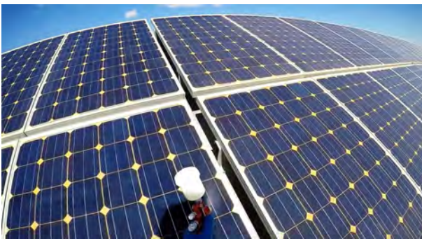
Picture 28 - Application of SurfaShield G on pre-installed panels
