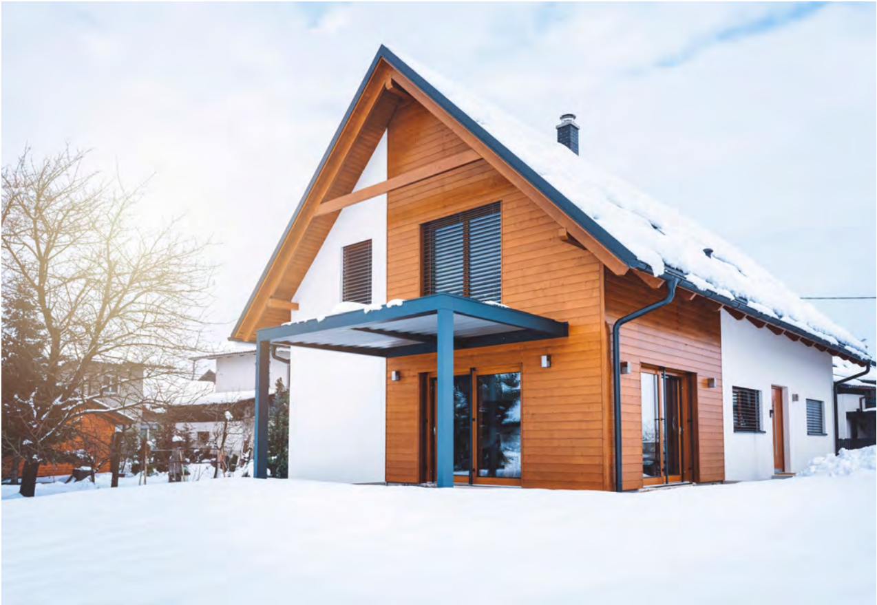
Picture 113 – Test application of both SurfaPaint Wood Arctic and SurfaPaint Wood Stain/Varnish-UV blocker in arctic conditions in Scandinavia
