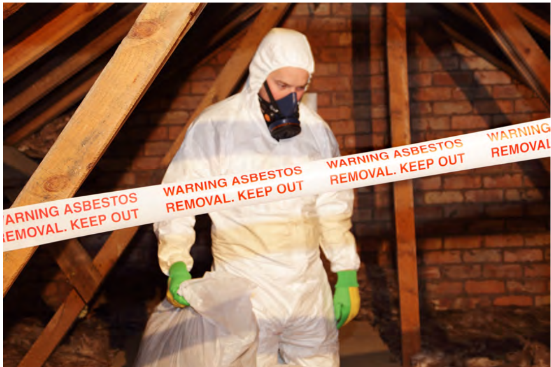
Picture 145 – Asbestos removal after stabilization with SurfaPore FX SB
