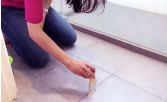
Picture 11 - Application of SurfaPore C on tile grout using a brush
