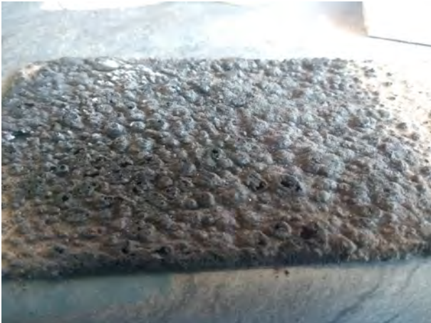
Picture 47 – SurfaPaint FireX Intumescent effect on a building surface
